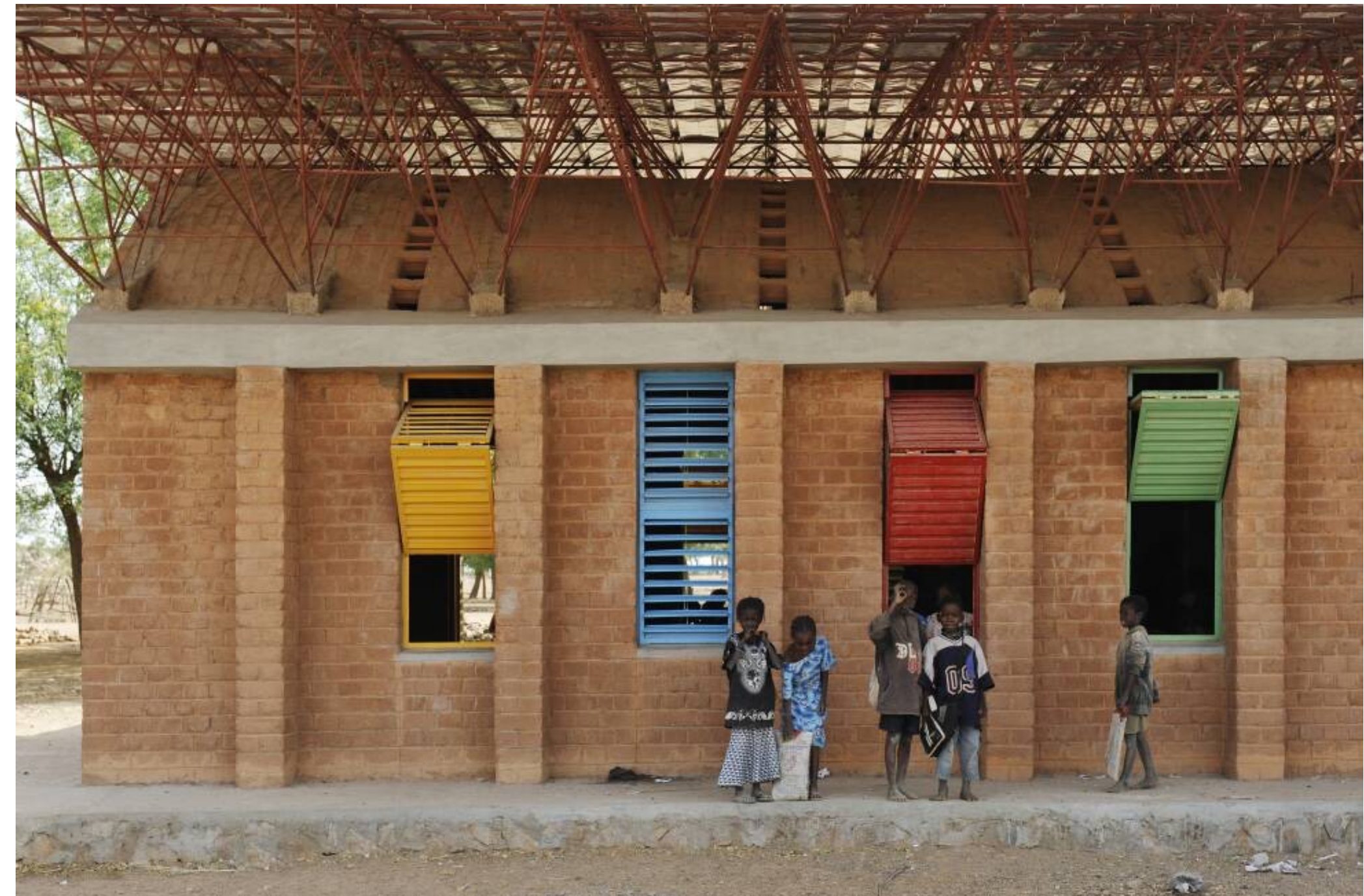
Gando Primary School Extension. Photo by Erik-Jan Ouwerkerk.
